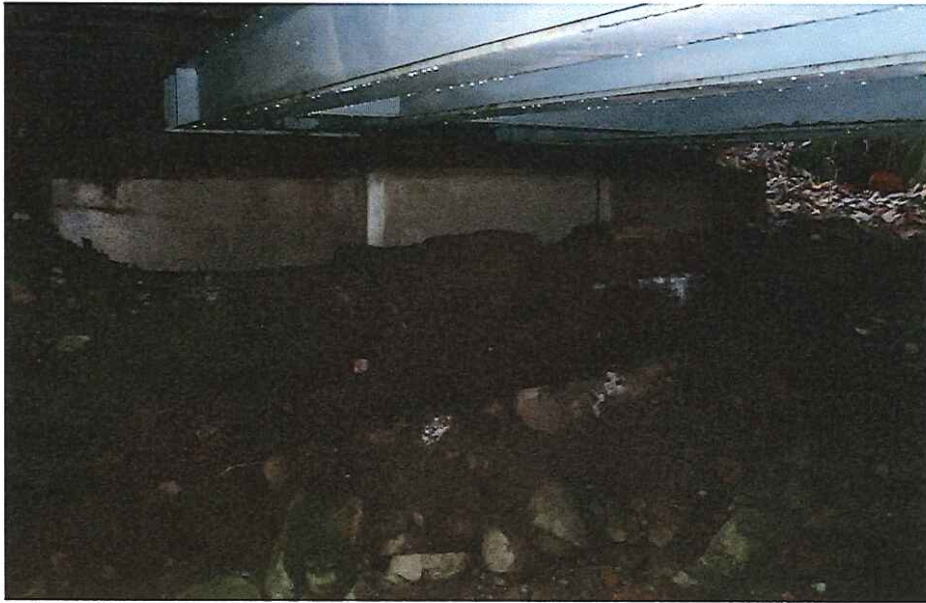
CK2011 Right Abutment
