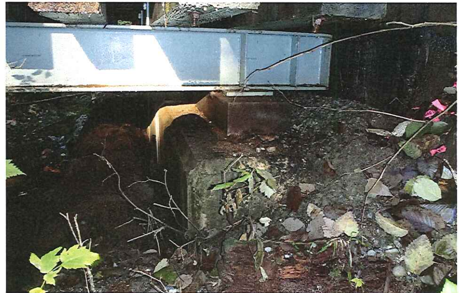
CK2011 Left Abutment bearing
