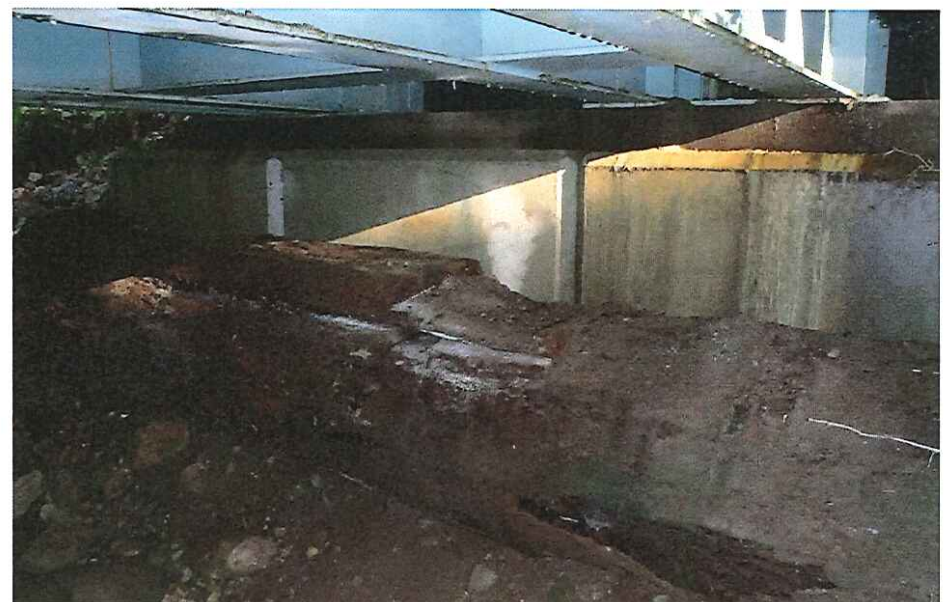
CK2011 Left Abutment
